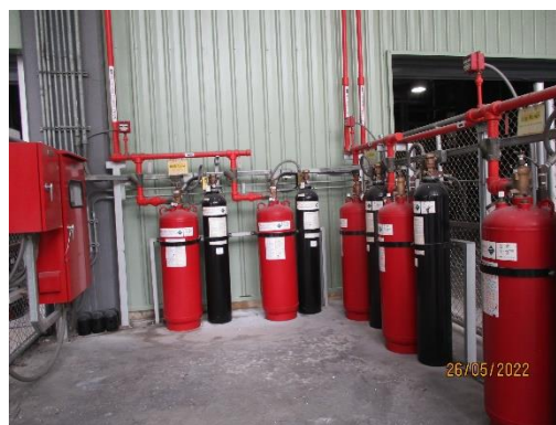
CO 2 Extinguishing Systems
