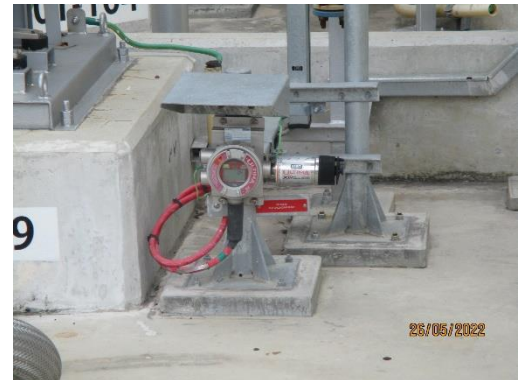
Flammable Gas Detectors
