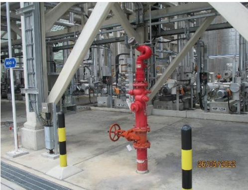
Fire Water Monitor with Foam Induction
