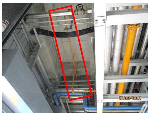
Automatic Foam Sprinkler System
