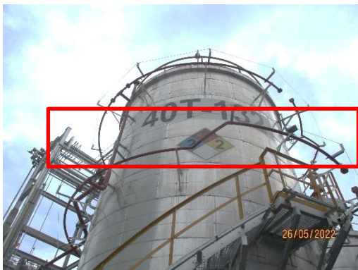
Automatic Water Sprinkler System
