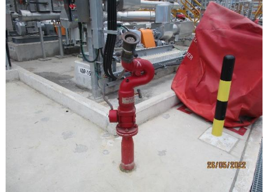
Fire Water Hydrants with Water Monitor
